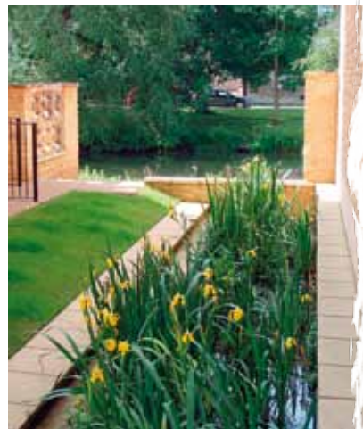
Riverside Court, Stamford – a canal as the final link in the management train, beginning with permeable paving, providing storage, amenity and biodiversity next to the River Welland. Photo: Bob Bray
