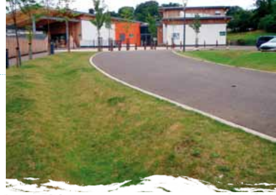
Exwick Heights School, Exeter – a shallow swale alongside the main access road into the school which begins the management train and leads to a wildlife pond. Photo: Bob Bray
