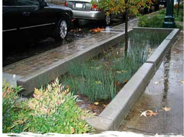
Portland, Oregon, USA – bioretention areas filter polluted road run-off, provide urban wildlife habitat and reduce local flooding. Photo: Dusty Gedge
