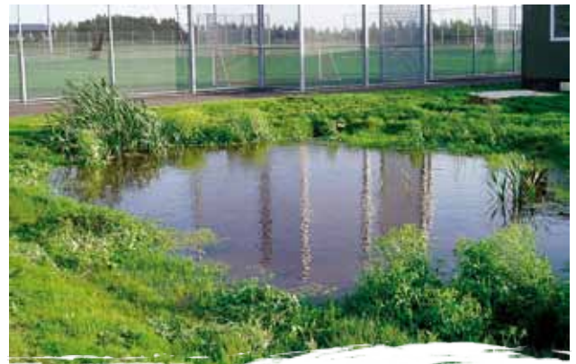
Pershore High School, Worcs – filter strips and swales play an important role intercepting silt, reducing flow rates and removing over 80% of pollution before allowing water to enter this pond. Photo: Bob Bray
