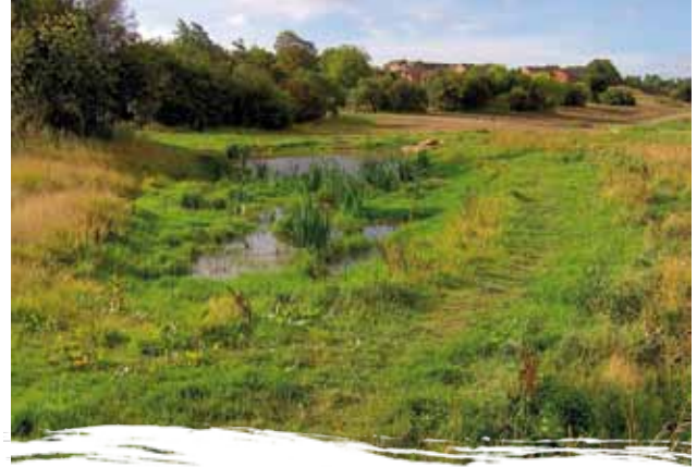
Manor Park, Sheffield – the third basin in the same scheme with a permanent pond and associated wet grassland habitat. Photo: Bob Bray
