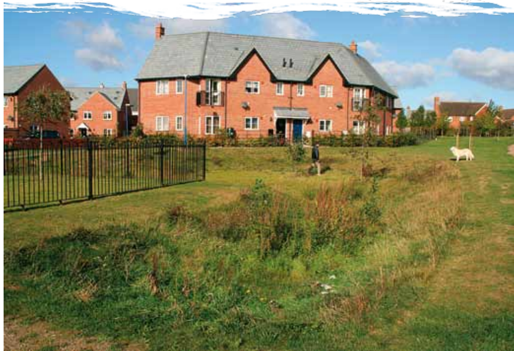
Lamb Drove, Cambourne – an open basin for occasional storage linked to a wet swale which is cut annually to enhance habitat whilst maintaining conveyance function. Photo: Bob Bray
