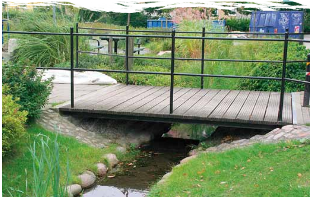
Augustenborg, Malmo, Sweden – an open grass and stone channel linking SuDS features and fully integrated into the landscape design. Photo: Bob Bray
