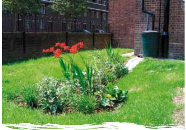
Ashby Grove Housing, Islington – a small urban rain garden demonstrating that any city green space can become a useful and attractive SuDS feature collecting roof water and protecting the sewer network. Photo: Jonathan Glerum (CIRIA)
