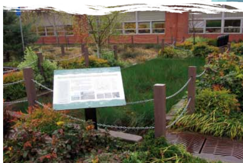
Portland, Oregon, USA – adaptation to climate change and extreme weather events are key services provided by SuDS. Photo: Dusty Gedge
