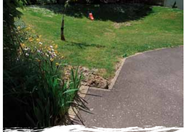
Springhill Housing, Stroud – a multi-functional detention basin and play space at the end of the management train that only fills after heavy rain. Photo: John Day (rspb)
