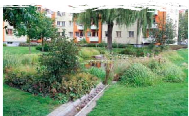
Augustenborg, Malmo, Sweden – an open channel leading from an unfenced amenity pond in a housing retrofit SuDS scheme. Photo: Bob Bray
